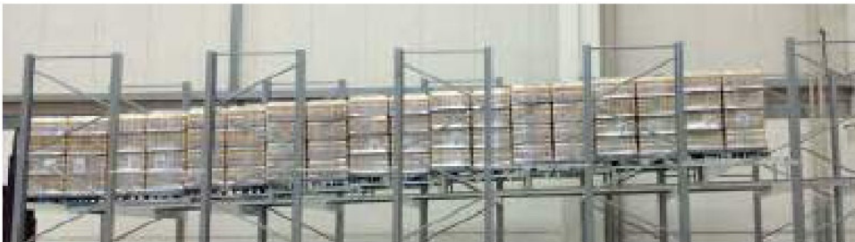
Magazzino in contropendenza LIFO attrezzato con moduli PUSH-BACK - LIFO warehouse with PUSH-BACK conveyors
