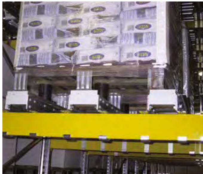
Modulo uscita con 3 piste a rulli per pallets Düsseldorf Unloading section with 3 roller tracks for pallets Düsseldorf
